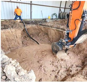
line is 15-17 feet deep and is a 21 or 24 inch main line. Mr. de Graffenried stressed that this is KWSC's repair, not the City of Lampasas's repair. Our utility employees are on site assisting and helping if needed. (Speculation is that the extreme heat may have caused subsurface movement.)
